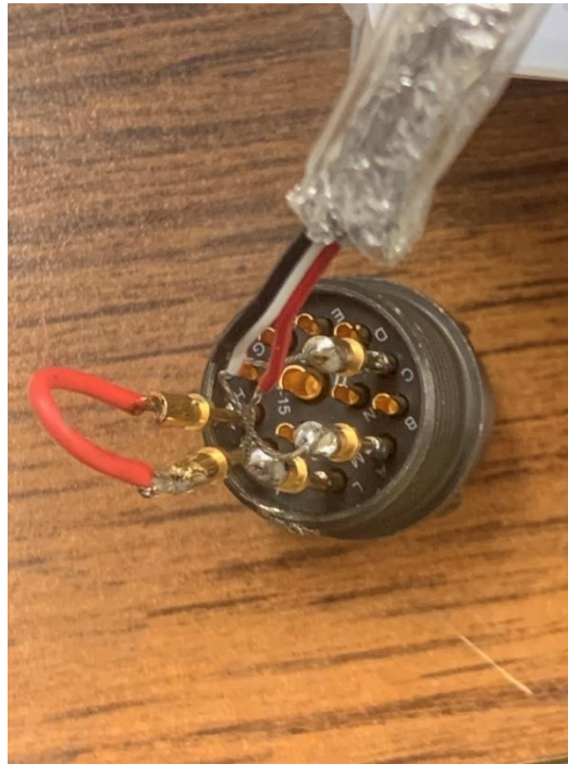
Fig. 3-7: The connection between the lead wires of the strain gauges and the input adaptor of the amplifier
