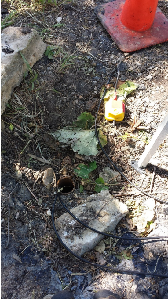
Figure 11. Surface geophone position next to the 5 ft (1.5 m) from the canal wall with downhole geophone cables.
