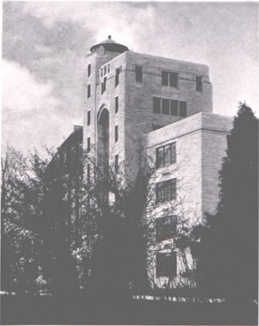
THE SCIENCE BUILDING
